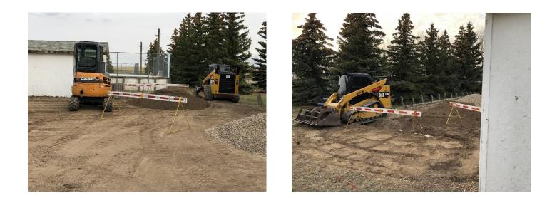
UPDATE APRIL 26, 2021 – Cypress County has completed the removal, re-fill and packing of the ground. ¾" crush has been spread on the site.
